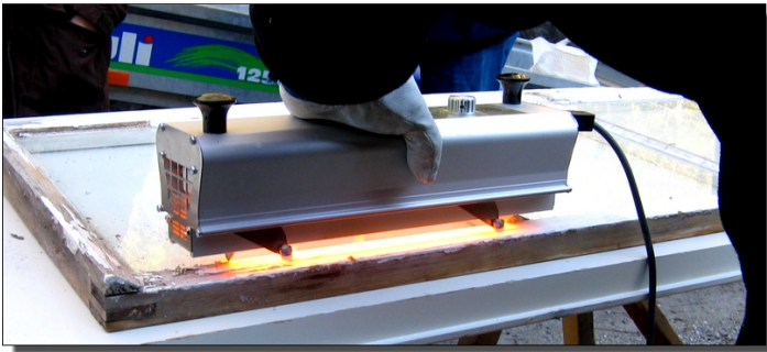
Old windowputty is being melted
