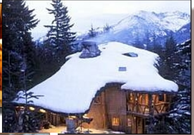
The generous eave overhangs keep the patio free from snow and give an inviting appearance.
